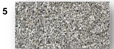
White Ballast Roof
